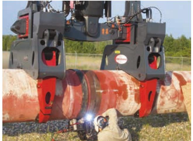
Figure 4. CRC-Evans tie-in station with weld positioner arms with M300-C mechanised welding system.
